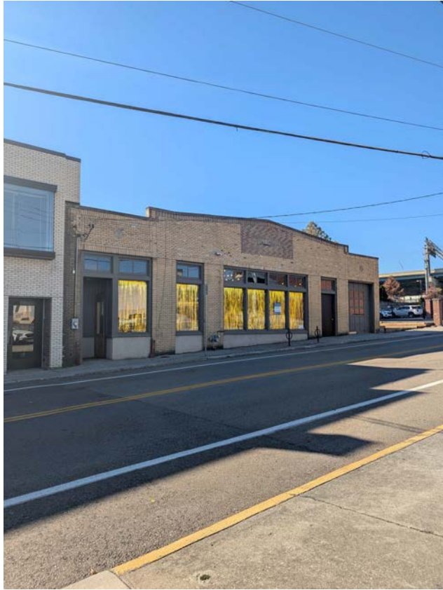
View Northwest From N. Central Street
