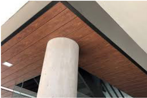
WOOD SOFFIT PANELS
