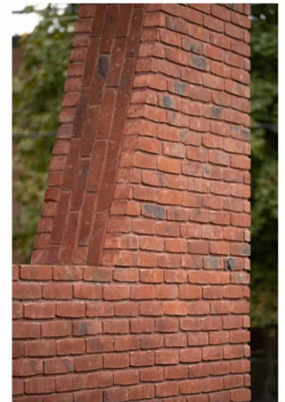
TAPERED BRICK COLUMN, TYPICAL
