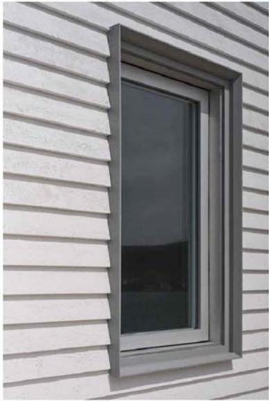
FIBER CEMENT TRIM 2" WINDOW JAMB PROJECTION
