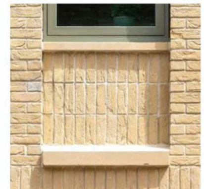
1/2" RECESSED BRICK UNDER WINDOW SILL
