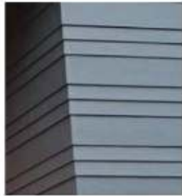
PAINTED FIBER CEMENT LAP SIDING WITH ALTERNATING EXPOSURES AND WOVEN CORNERS
