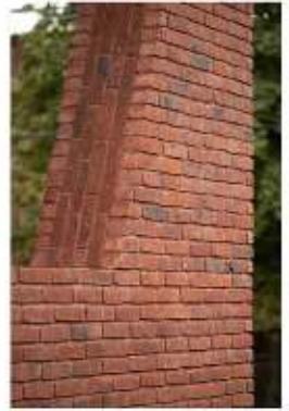
TAPERED BRICK COLUMN, TYPICAL
