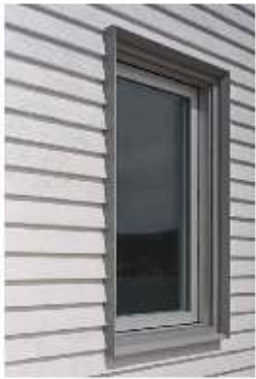
FIBER CEMENT TRIM 2" WINDOW JAMB PROJECTION
