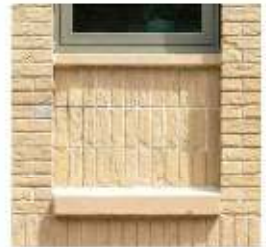
1/2" RECESSED BRICK UNDER WINDOW SILL
