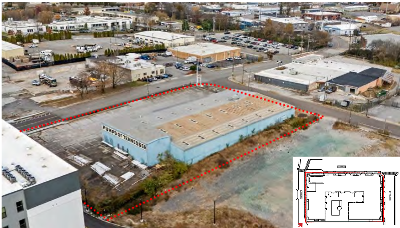
Along Florida St. facing North
