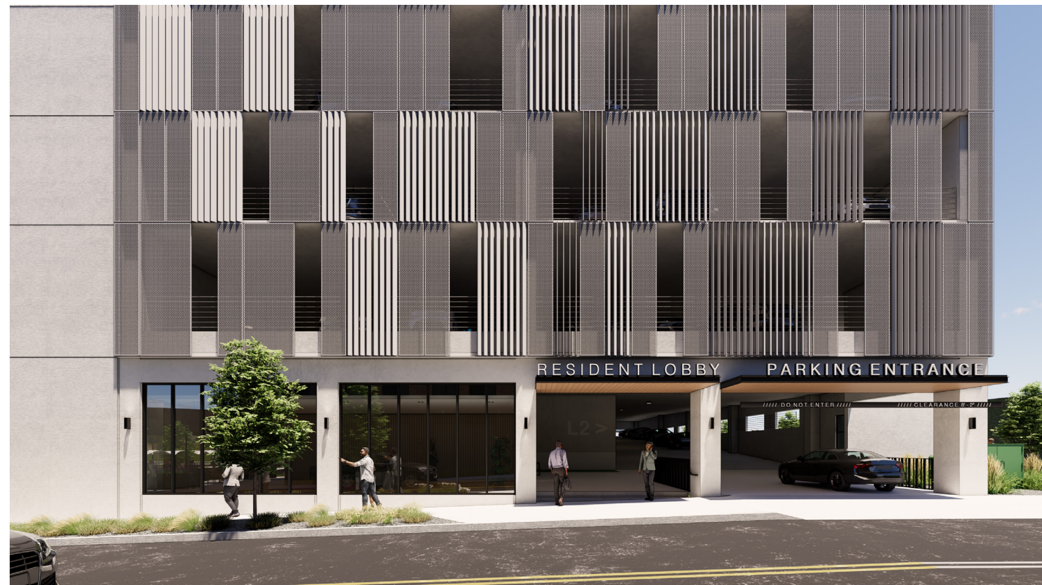
PARKING GARAGE ENTRY OFF MORGAN ST.
