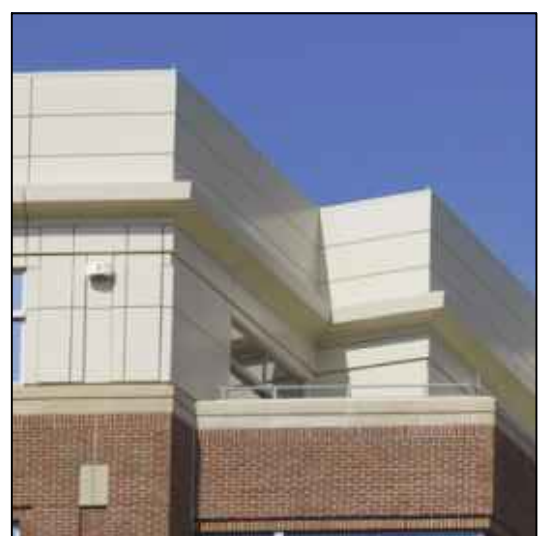
NEW OPERABLE WINDOW UNIT, COLOR TO MATCH WINDOW STOREFRONT COLOR CONCEALED FASTENER METAL PANEL
