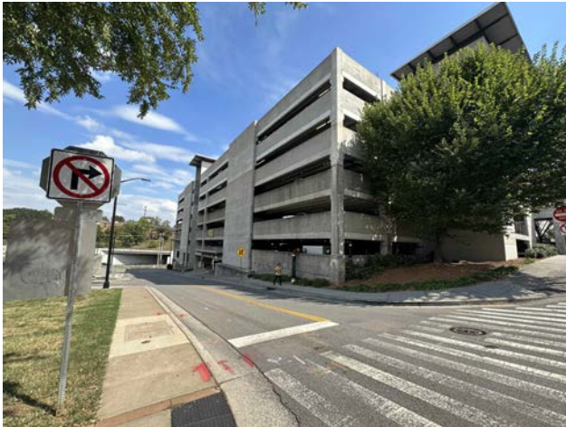
VIEW LOOKING SOUTH
