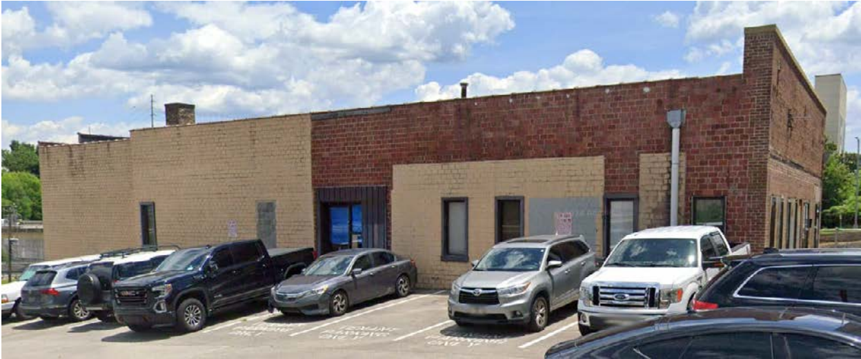
This view shows the side of the building from Cumberland Ave.
