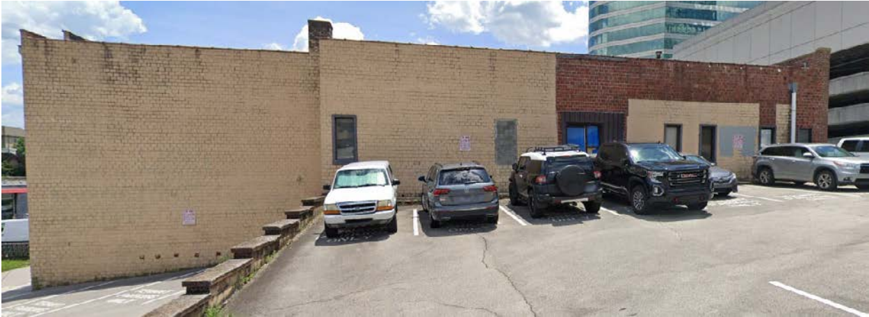
This picture shows the side of the building from Cumberland Ave, and the other parking lot that will be remarked.
