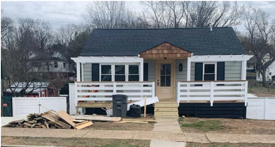
Porch addition as completed
