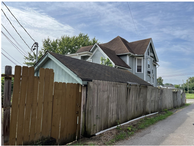
SHED AND FENCE TO BE REMOVED
