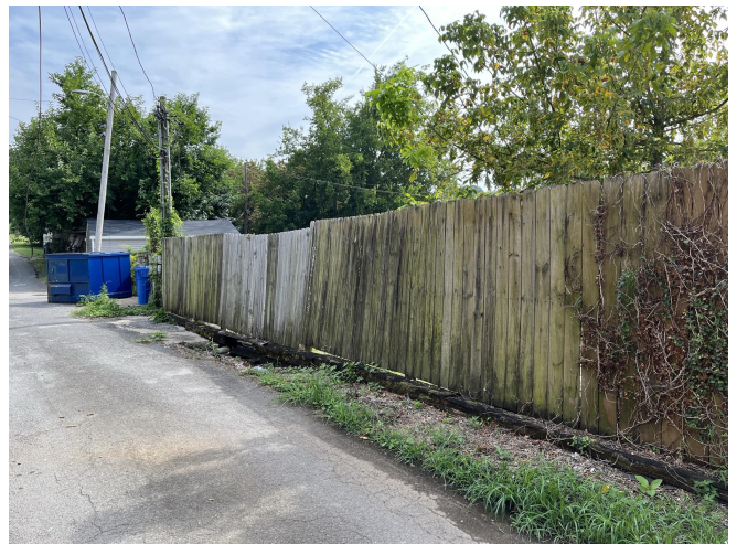
FENCE TO BE REMOVED
