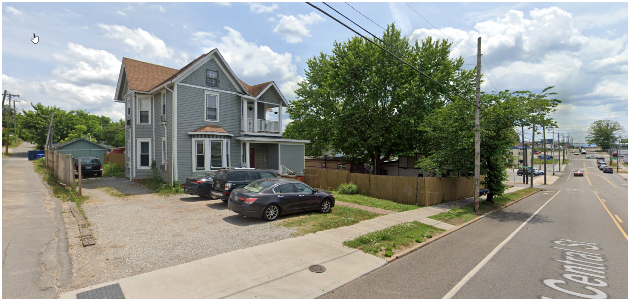
VIEW FROM GOOGLE STREET VIEW DATED 2021 - N CENTRAL ST AND OLDHAM AVE
