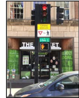
SIGNAL #11 SOUTHEAST CORNER ORIGINAL POLE IDENTIFICATION: TM1.4 ORIGINAL FOUNDATION TYPE: TM-3 ORIGINAL POLE DETAIL TYPE: 3L NOTE: INCLUDE SUPPLEMENTAL SIGNAL HEAD TO ATTACH TO NEW POLE.
