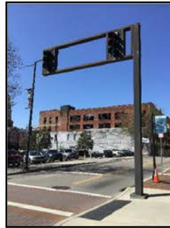
SIGNAL #5 NORTHWEST CORNER ORIGINAL POLE IDENTIFICATION: TM-D ORIGINAL FOUNDATION TYPE: TM-4, ORIGINAL POLE DETAIL TYPE: NA
