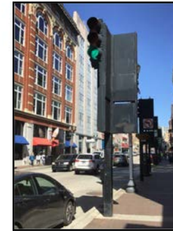
SIGNAL #11 SOUTHEAST CORNER ORIGINAL POLE IDENTIFICATION: TM1.4 ORIGINAL FOUNDATION TYPE: TM-3 ORIGINAL POLE DETAIL TYPE: 3L NOTE: INCLUDE SUPPLEMENTAL SIGNAL HEAD TO ATTACH TO NEW POLE.
