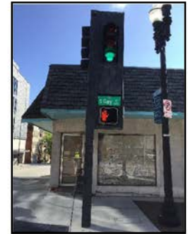
SIGNAL #2 SOUTHEAST CORNER ORIGINAL POLE IDENTIFICATION: TM-B ORIGINAL FOUNDATION TYPE: TM-3 ORIGINAL POLE DETAIL TYPE: 2
