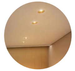
DOWNLIGHTING - UNDER MEZZANINE
