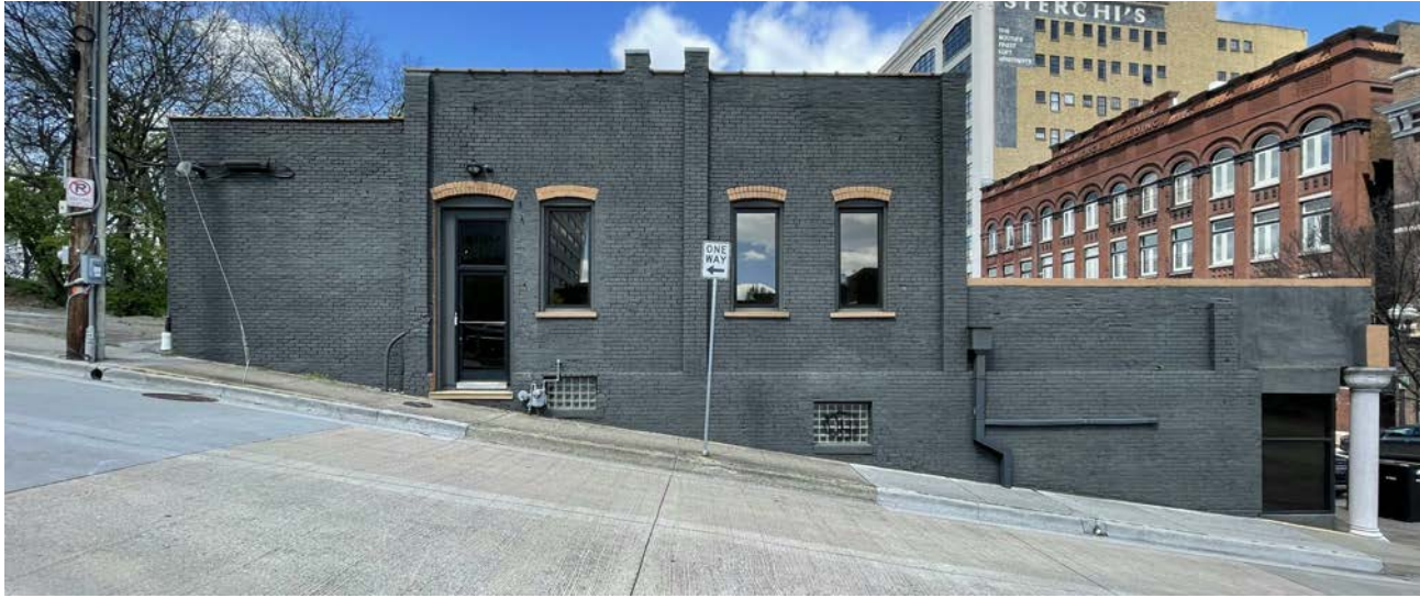
K21 SOUTHEAST ELEVATION NOT TO SCALE EXISTING PHOTO
