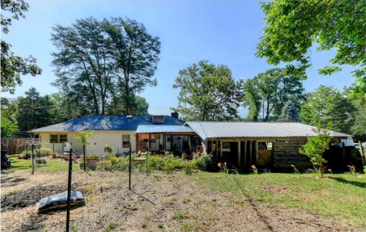
Rear facades of structures prior to fire.
