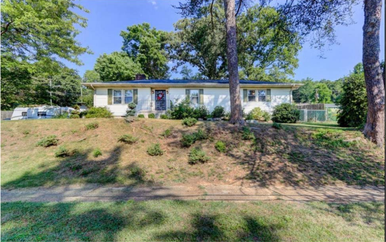
Front façade of house (garage view obscured by RV).
