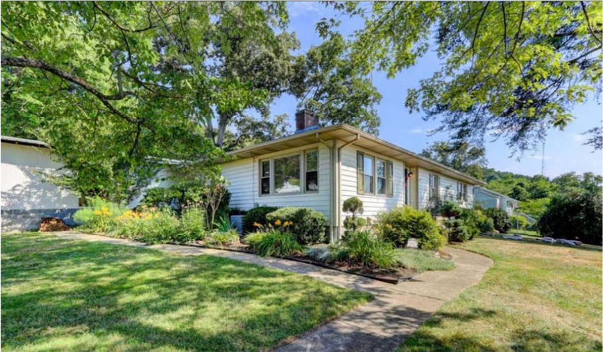
View of corner where house and garage roofs will meet.
