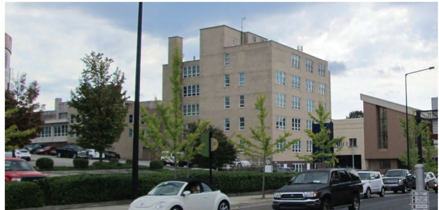
EXISTING BUILDING _ NORTHWEST CORNER FROM HENLEY ST
