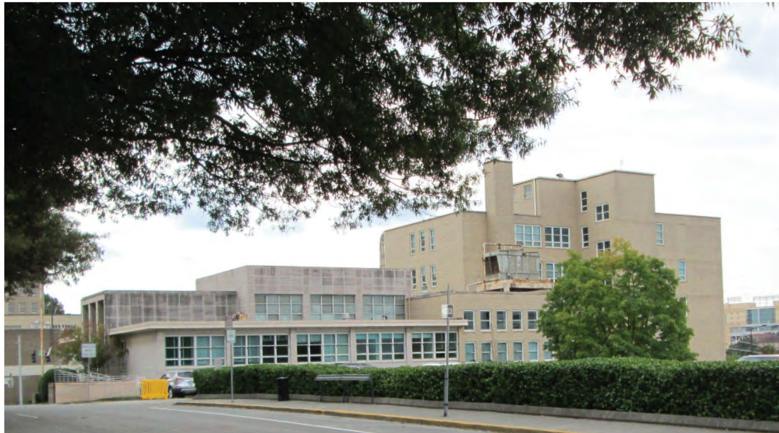
EXISTING BUILDING _ NORTH ELEVATION FROM LOCUST ST
