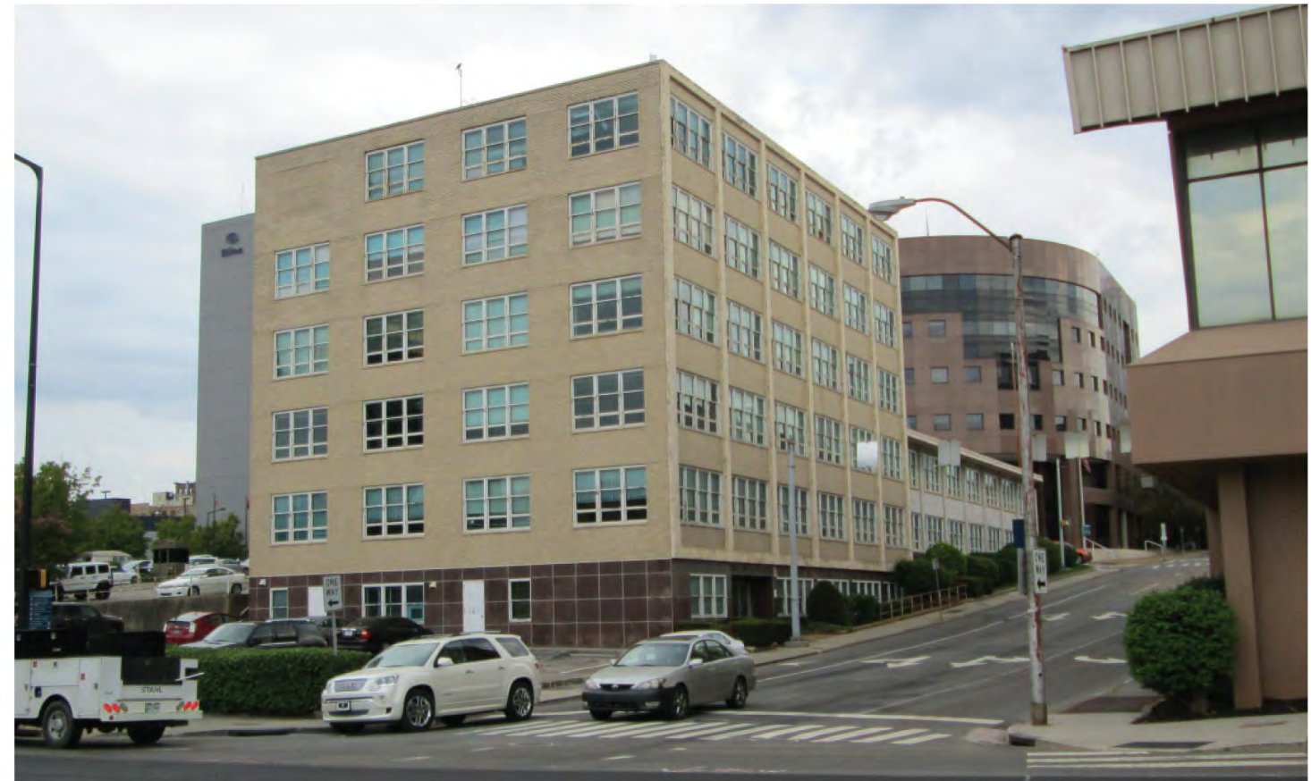
EXISTING BUILDING _ SOUTHWEST CORNER FROM CUMBERLAND AVE & HENLEY ST INTERSECTION
