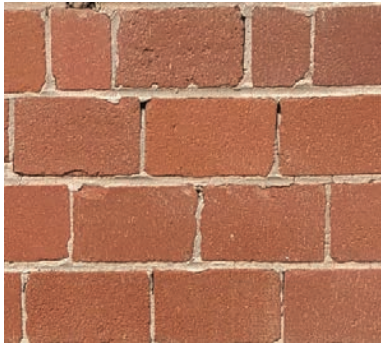
EXISTING TERRACOTTA BLOCK
