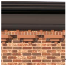
Decorative Cornice Painted Sherwin Williams Black Fox
