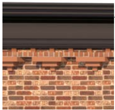
Decorative Cornice Painted Sherwin Williams Black Fox
