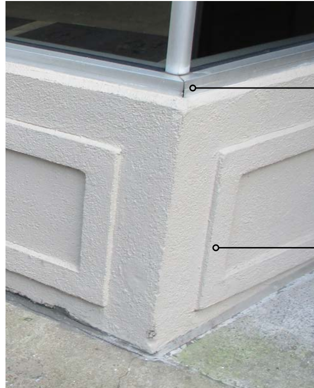
ALUMINUM STOREFRONT WINDOW TO BE REMOVED
