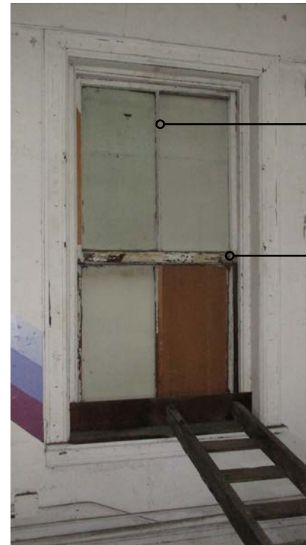
PLYWOOD INFILL PANEL AT DAMAGED WINDOW TO BE REMOVED
