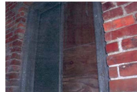
WINDOWS INFILLED FROM INTERIOR AT FIRST LEVEL
