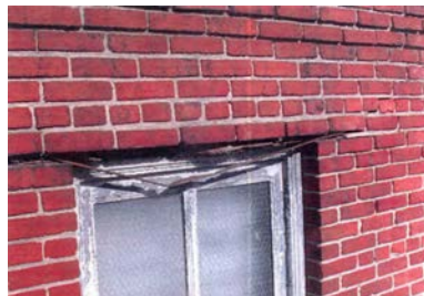
FAILED STEEL LINTELS
