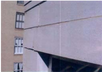
STONE ABOVE LINTELS HAS SHIFTED AND NEEDS REPAIR
