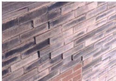
FAILED STEEL LINTELS
