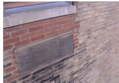
INFILL AT GRILL AND STEP CRACK IN BRICK BELOW
