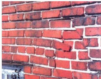
BRICK FACES SHEARED AT STEP CRACK
