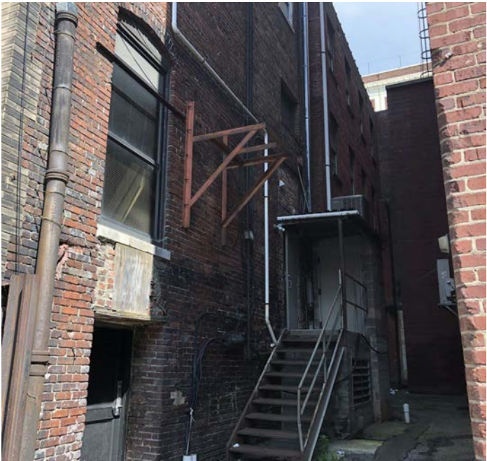
STONE ABOVE LINTELS HAS SHIFTED AND NEEDS REPAIR
