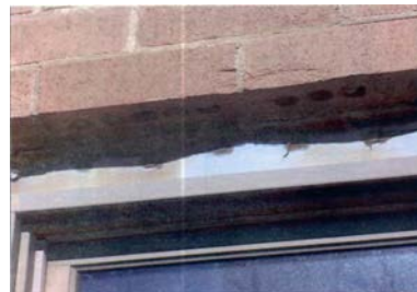
PARTIALLY INFILLED WINDOWS- NO LINTEL
