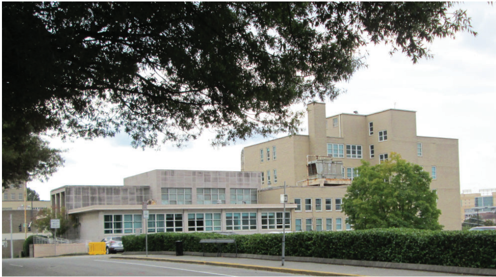
EXISTING BUILDING _ NORTH ELEVATION FROM LOCUST ST
