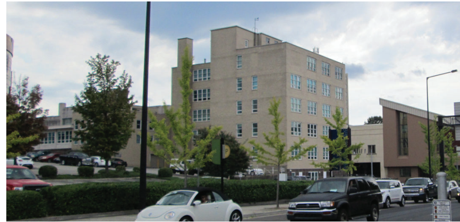
EXISTING BUILDING _ NORTHWEST CORNER FROM HENLEY ST
