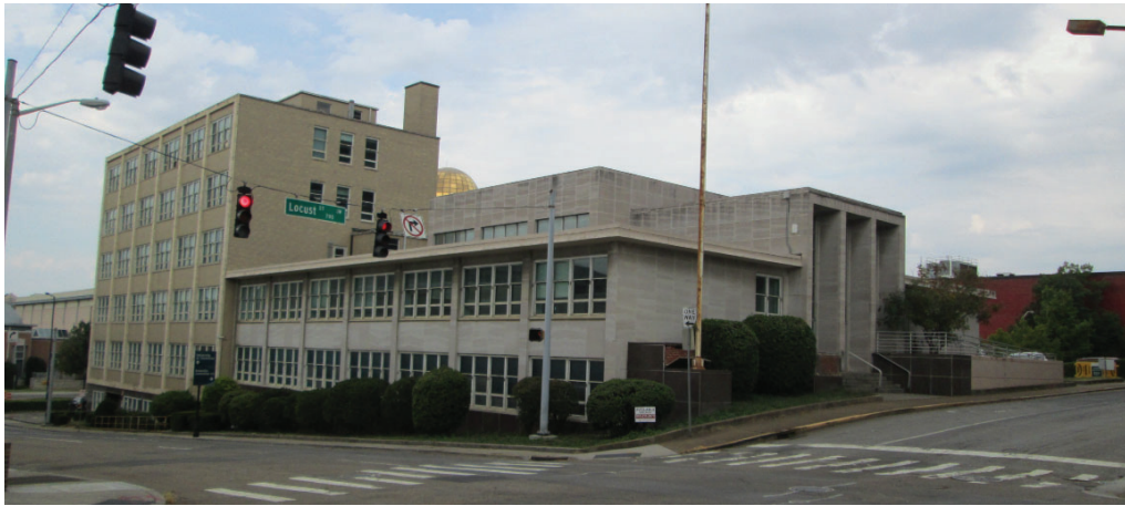
EXISTING BUILDING _ SOUTHEAST CORNER FROM CUMBERLAND AVE & LOCUST ST INTERSECTION
