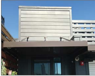
PREFINISHED ALUMINUM CANOPY, PAINTED CEMENT BOARD SIDING
