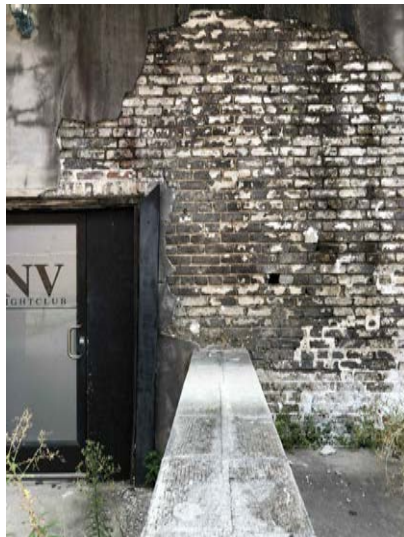
Existing Brick - Exposed Condition
