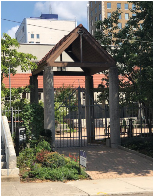
EXISTING COURTYARD PORTAL
