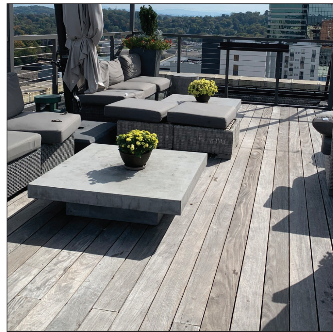
IPE WOOD DECKING, FURNITURE AND CABLE RAIL
