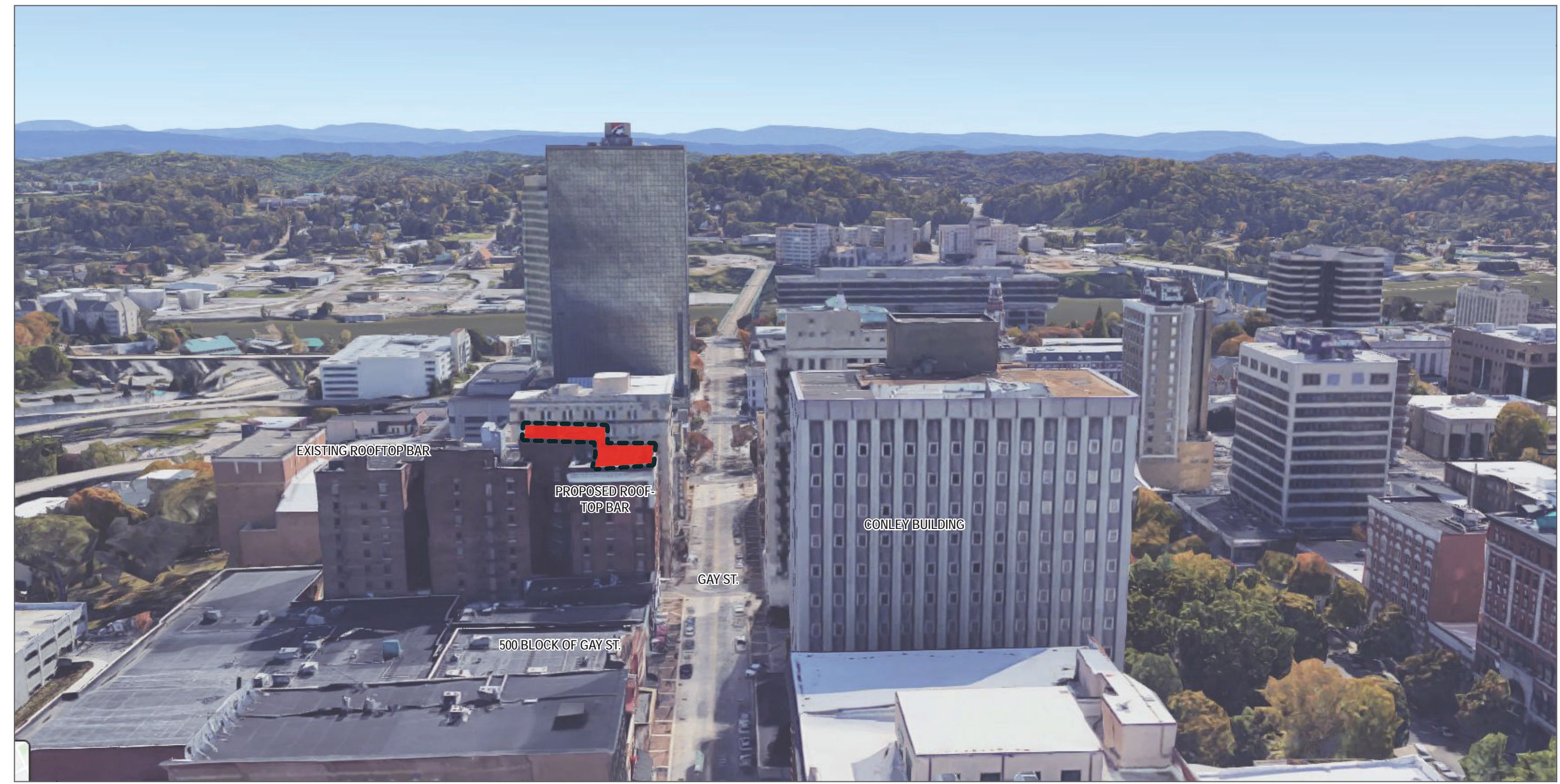
AERIAL VIEW LOOKING SOUTH
