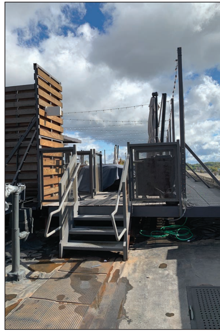
EXISTING ROOFTOP LOOKING WEST
