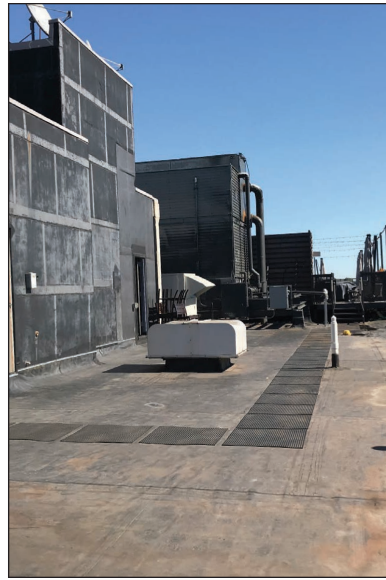
EXISTING ROOFTOP LOOKING WEST
