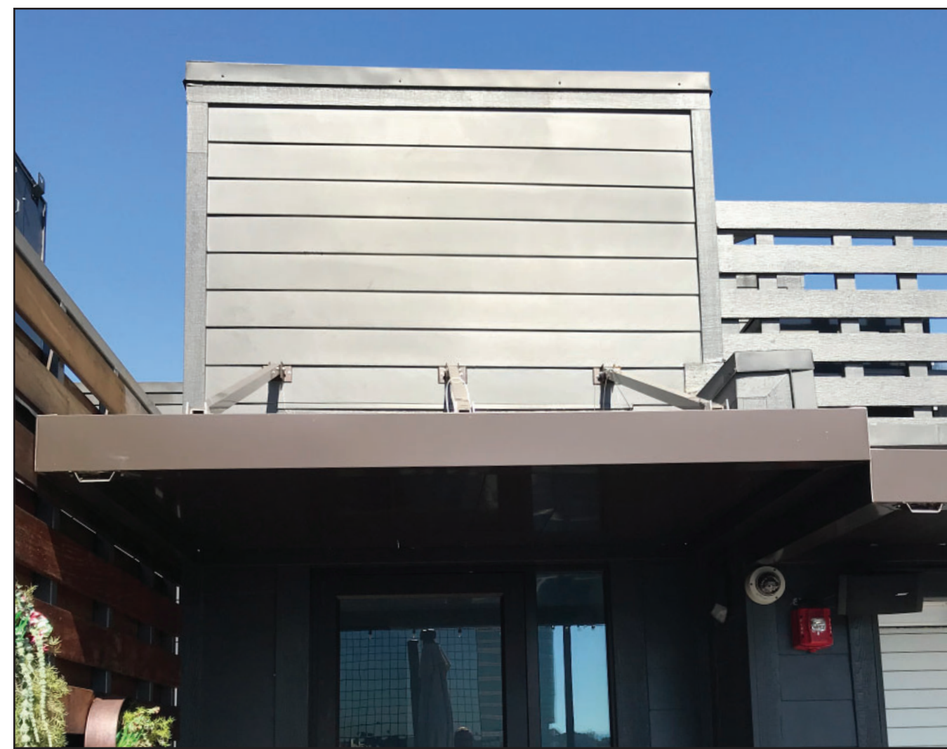
PREFINISHED ALUMINUM CANOPY, PAINTED CEMENT BOARD SIDING
