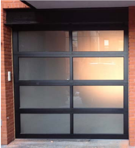
SEGMENTAL OVERHEAD ALUMINUM DOOR WITH GLAZED PANELS WITH TRANSLUCENT FILM APPLIED TO GLASS
