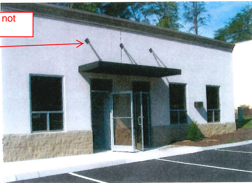
Similar canopy installation by Rusco Custom Canopies
