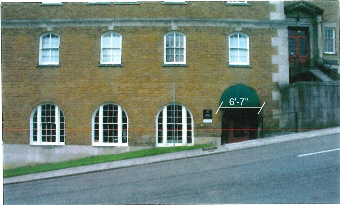
East elevation- First Baptist Church facing Locust Street and City/County Building
