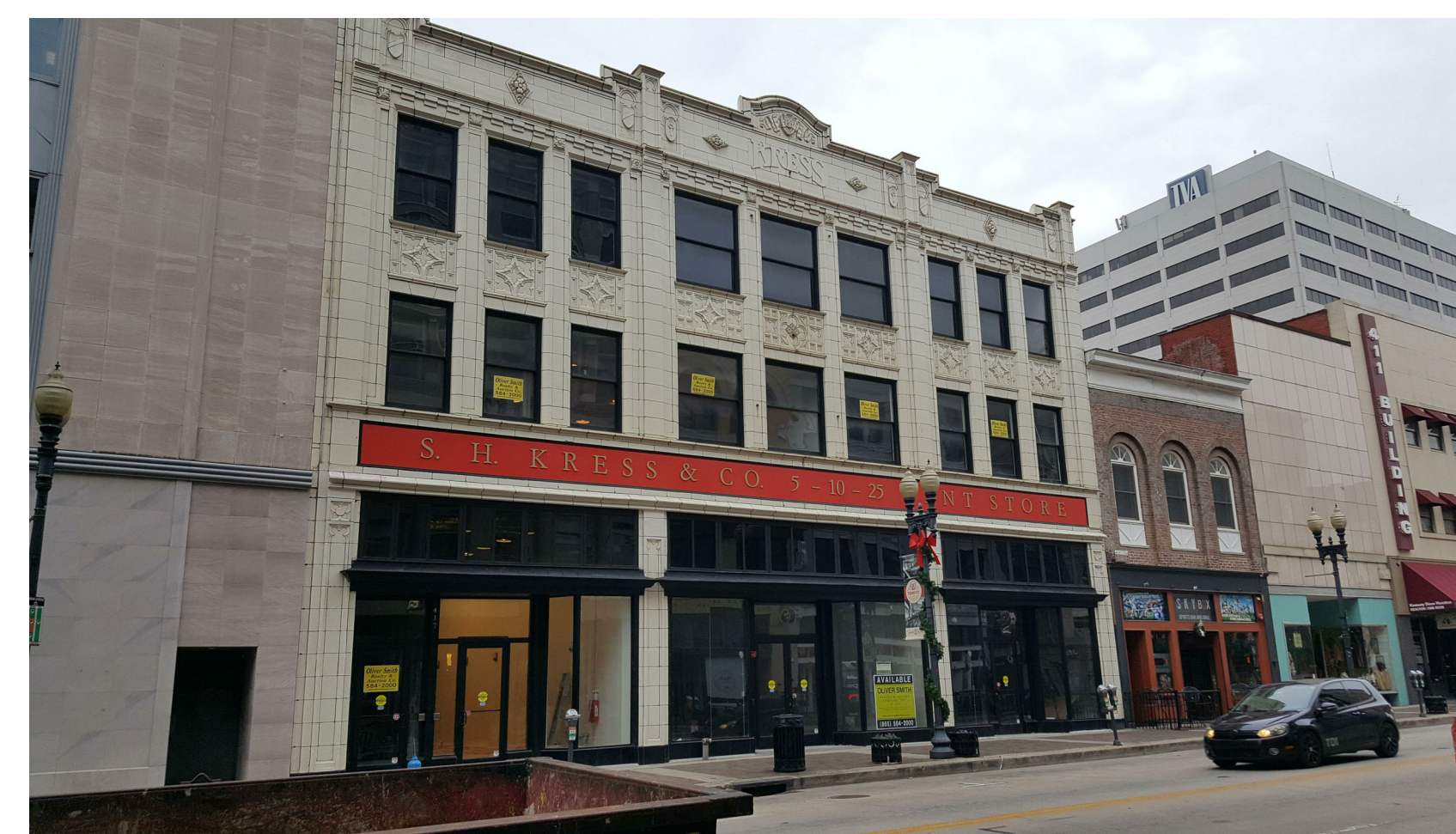
PHOTO OF THE EXTERIOR OF THE KRESS BUILDING, 417, 419, 421, AND 423 GAY STREET
