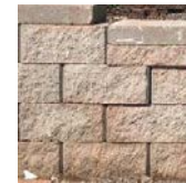
Segmented Block Retaining Wall
