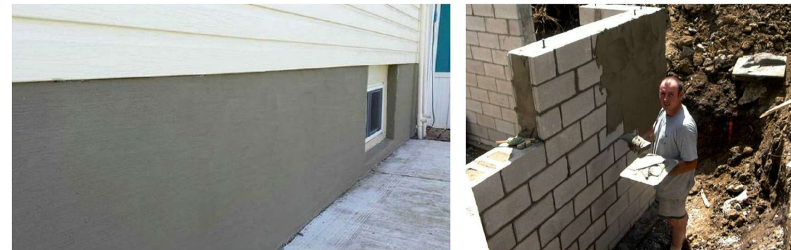
Examples of parged CMU walls.
