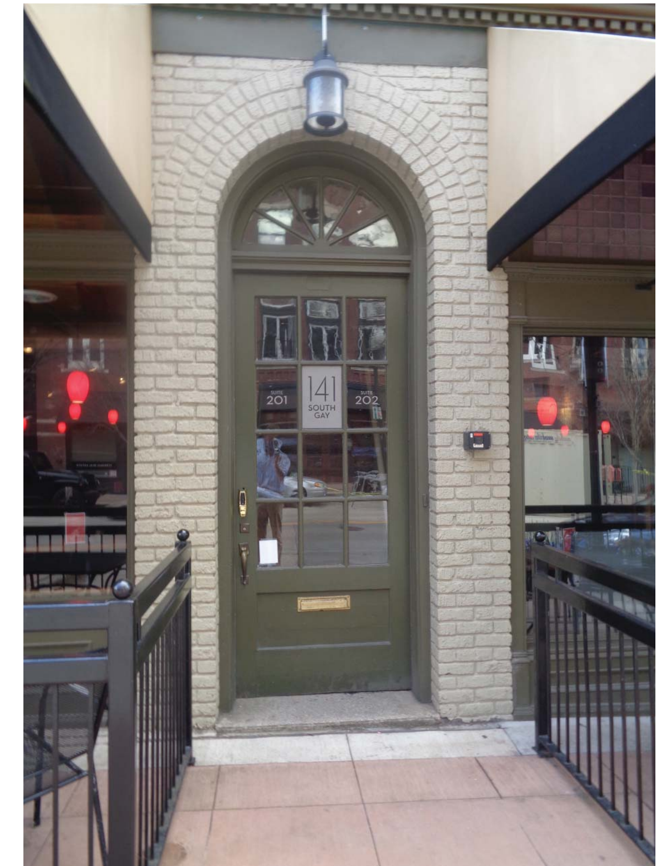
ENTRANCE TO APTS. FROM GAY STREET - NO WORK PLANNED
