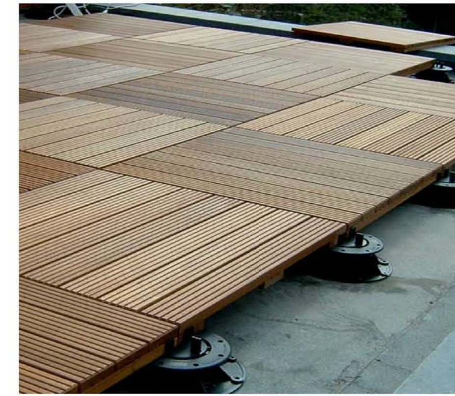
MODULAR WOOD DECKING ON PEDESTAL SYSTEM
