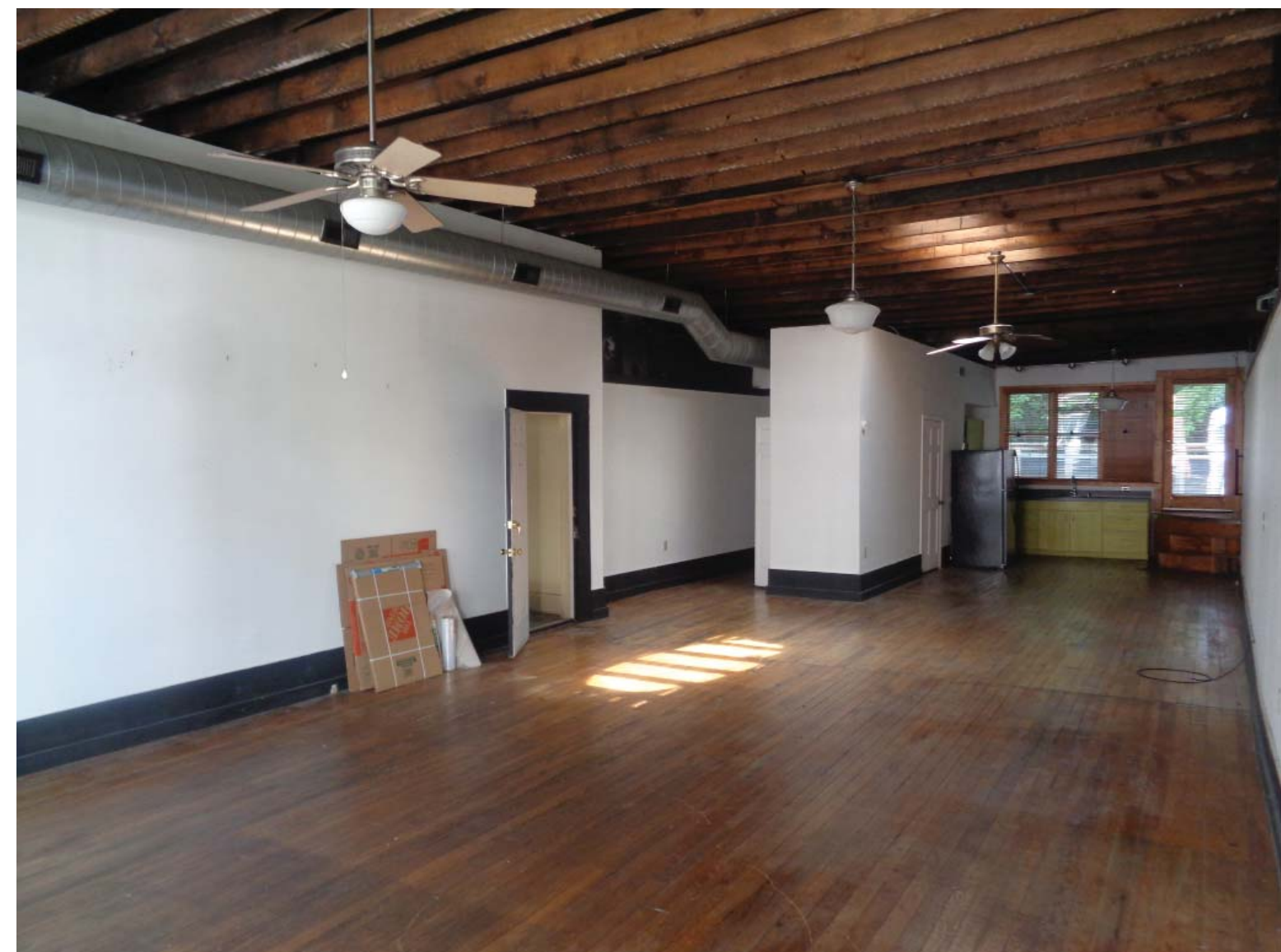
EXISTING INTERIOR OF APARTMENT 202. LOOKING WEST.
