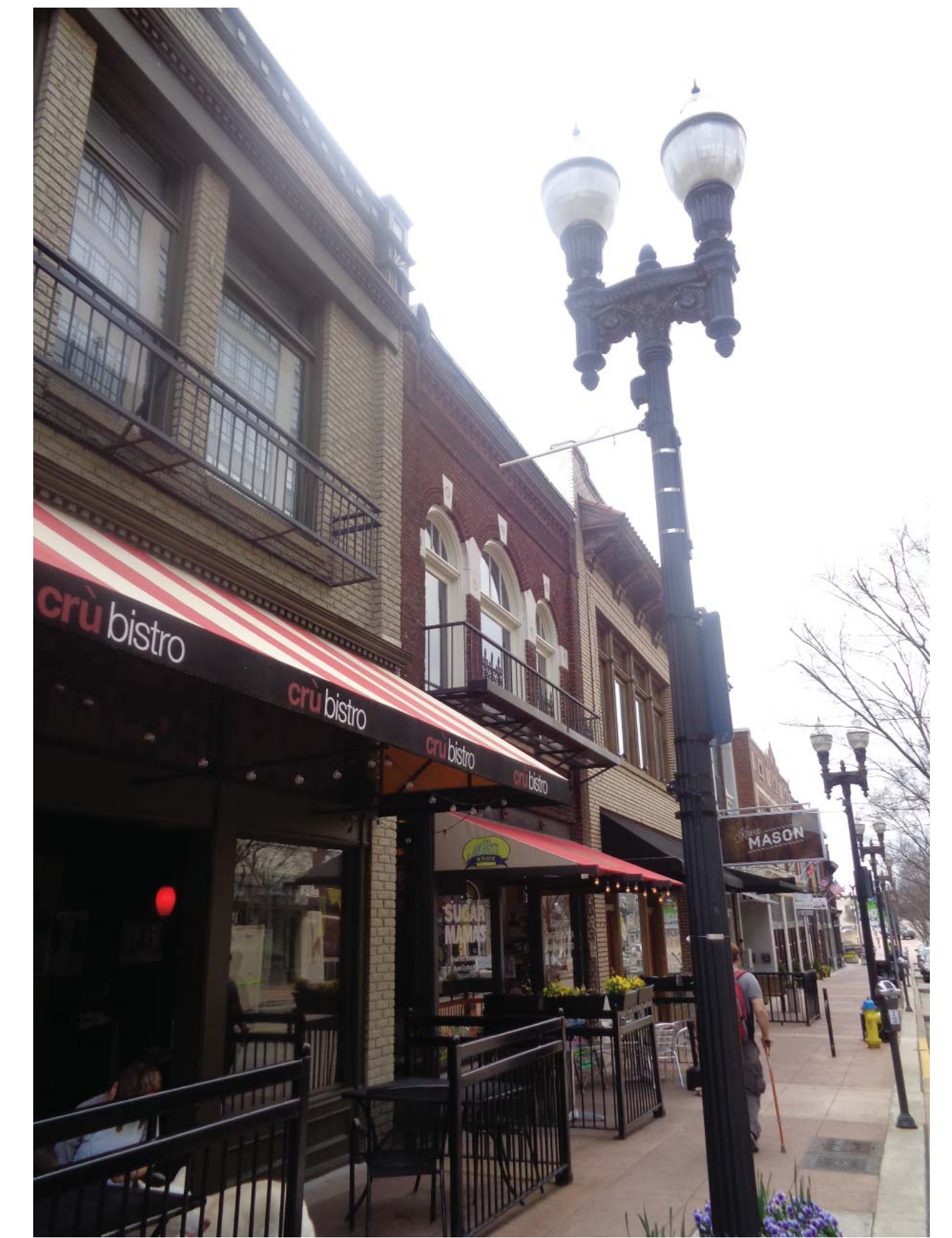
VIEW FROM GAY STREET. APT 202 IS ABOVE AWNING - NO WORK PLANNED
