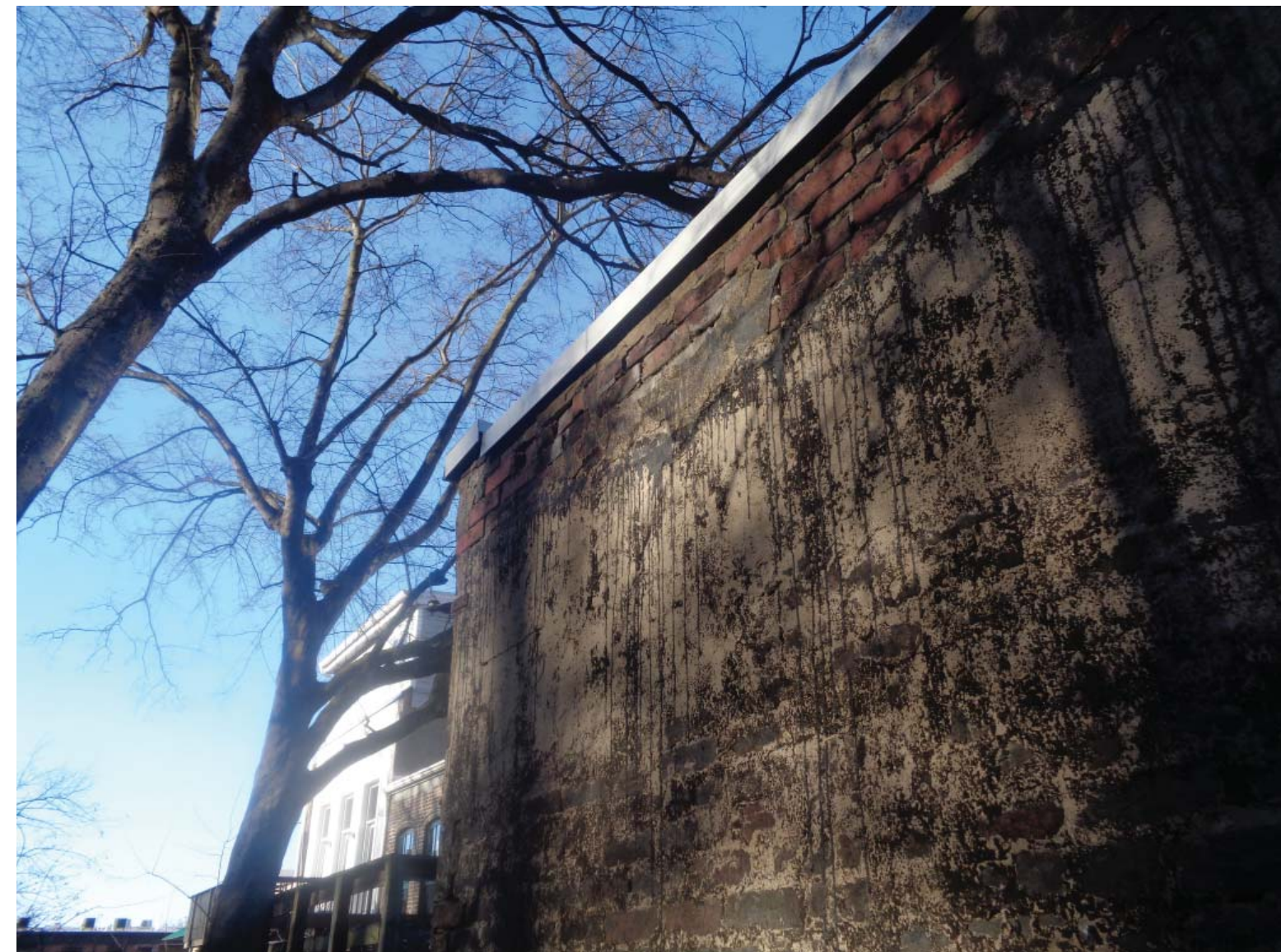
EXISTING WEST WALL OF STORAGE ROOM - BRICK JOINTS WILL BE REPOINTED AS REQ.
