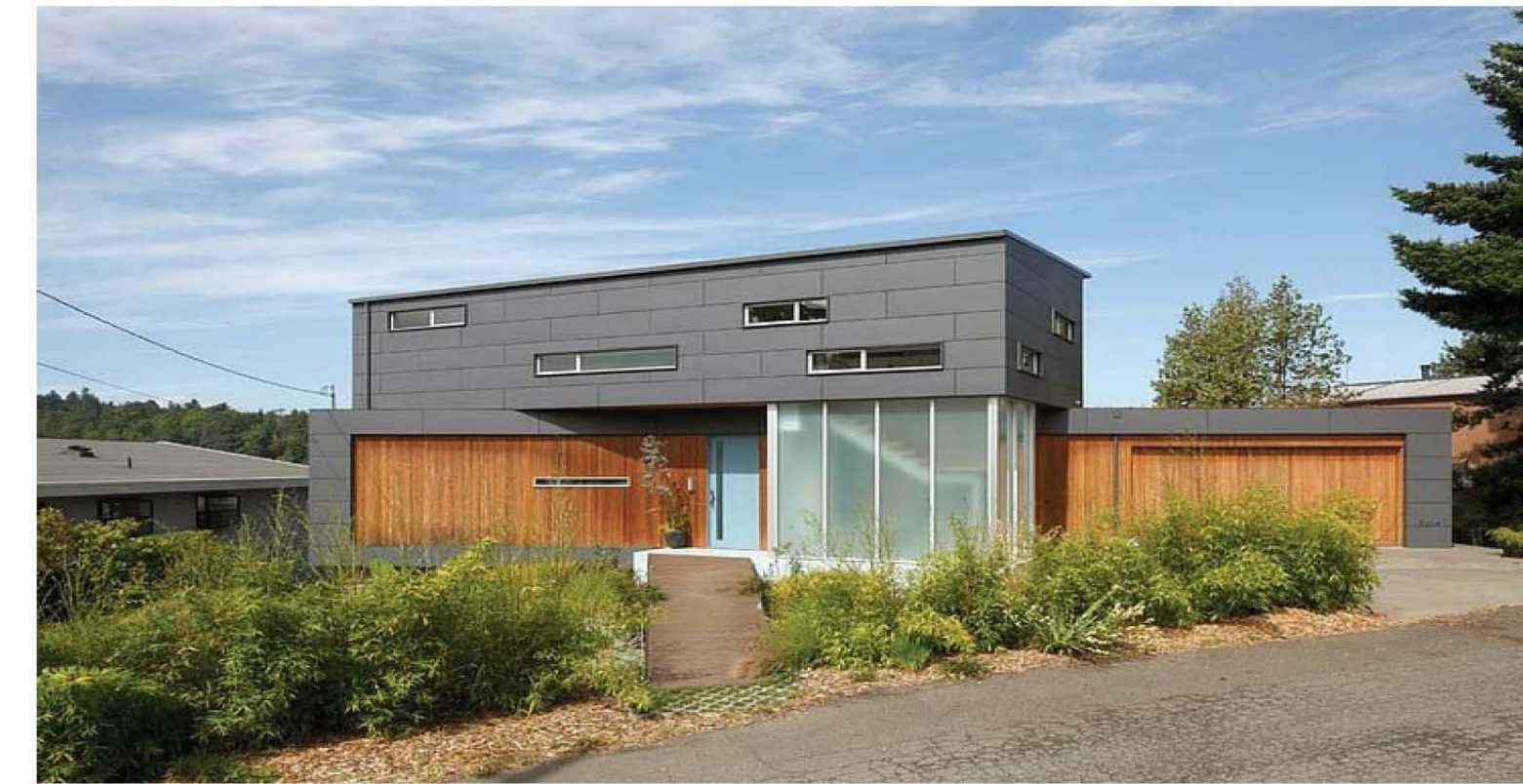
PAINTED CEMENT BOARD SIDING WITH REVEALS
