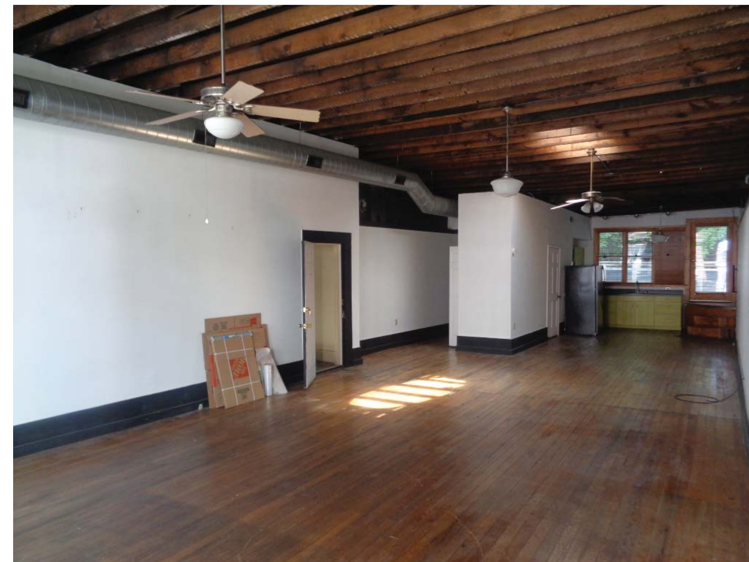
EXISTING INTERIOR OF APARTMENT 202. LOOKING WEST.
