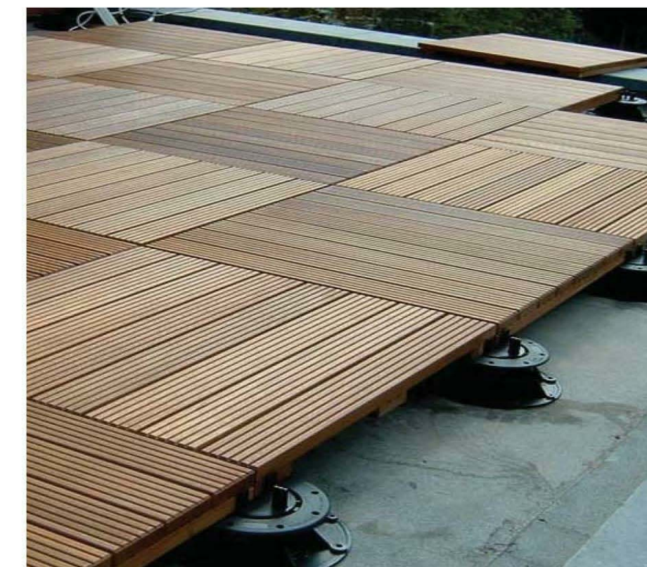
MODULAR WOOD DECKING ON PEDESTAL SYSTEM
