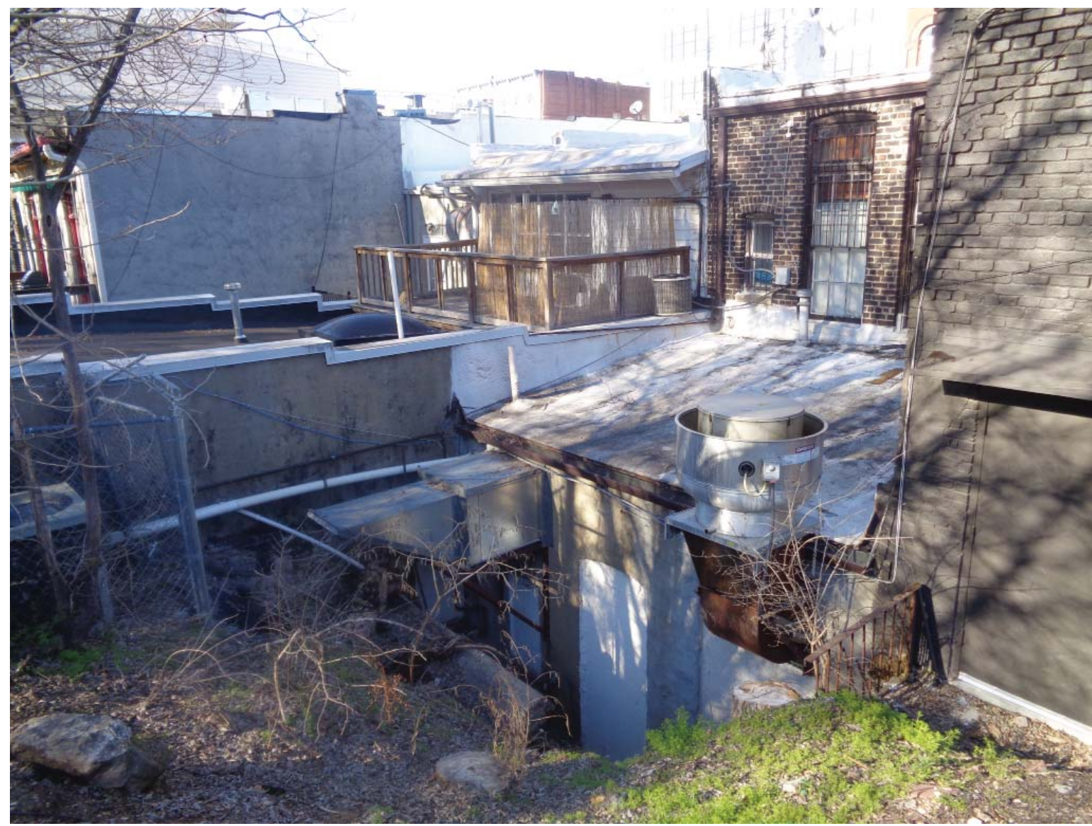
EXISTING STORAGE ROOM AND KITCHEN. APARTMENTS 201 AND 202 ABOVE.
