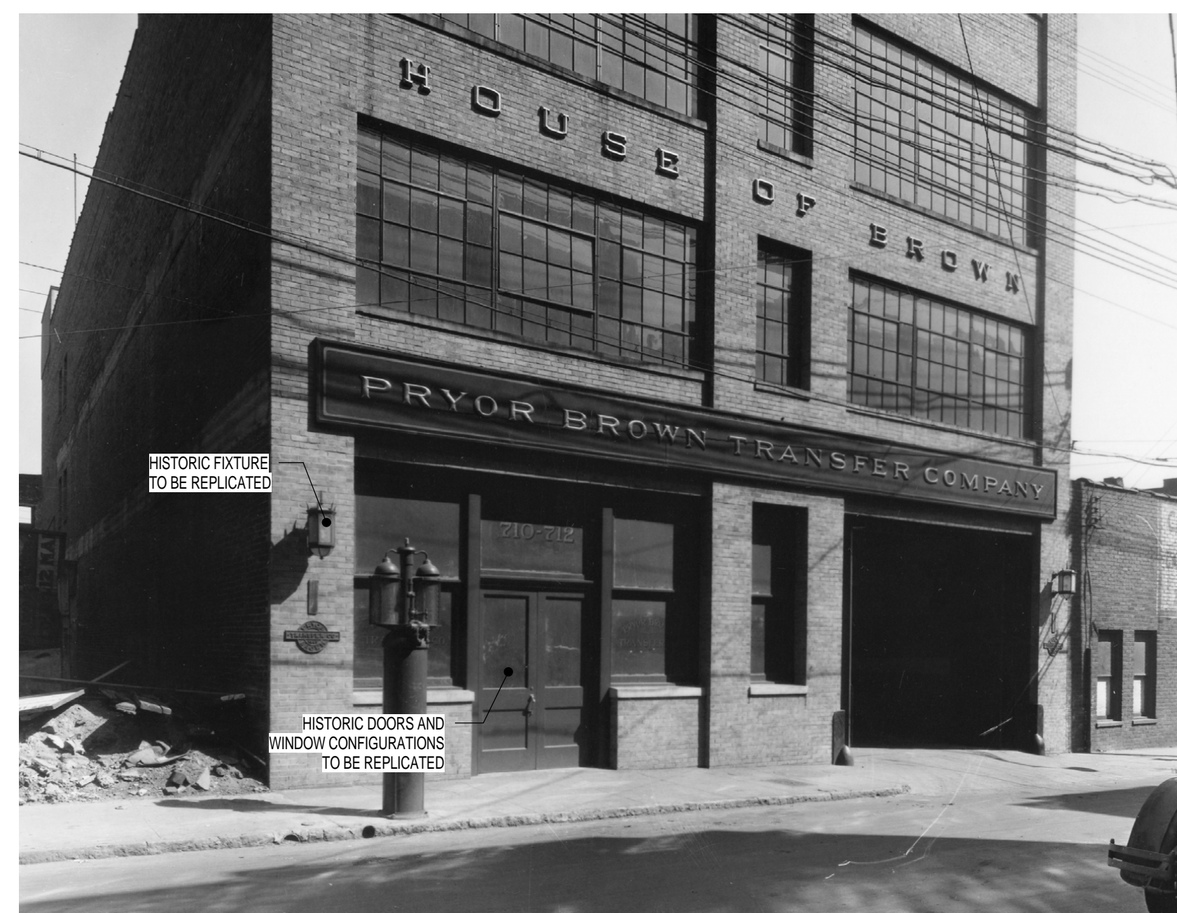
VIEW AT MARKET STREET OF SOUTHERN PORTION OF ORIGINAL BUILDING
