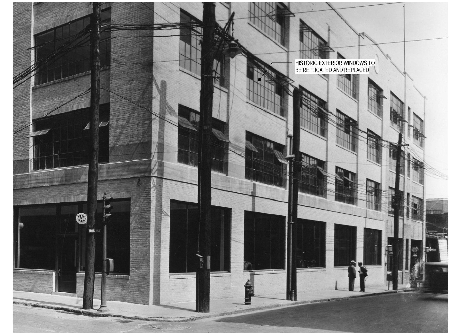
VIEW AT MARKET STREET
