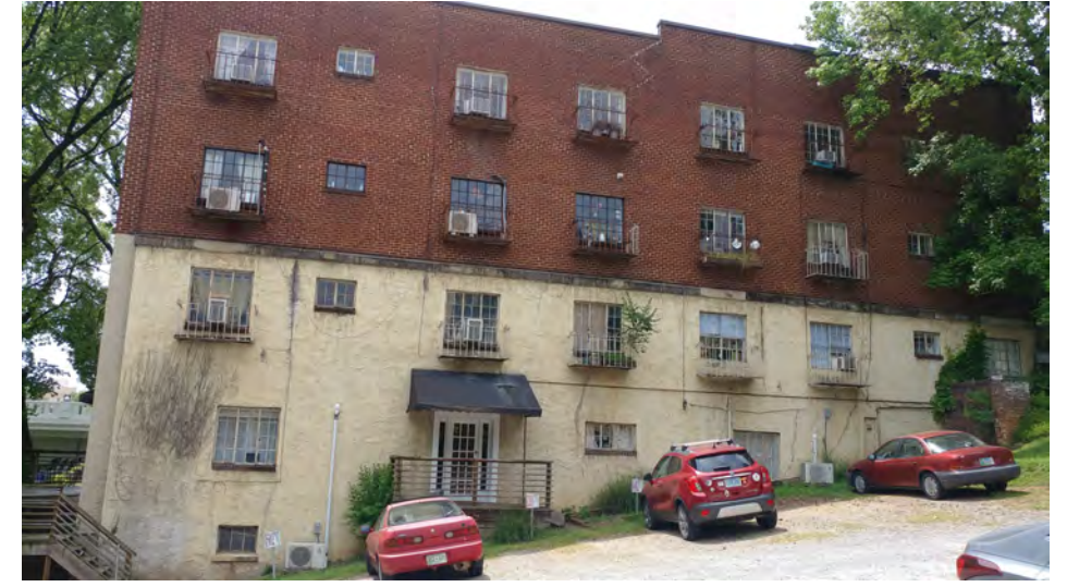
2 FROM SITE LOOKING AT RIVERHOUSE
