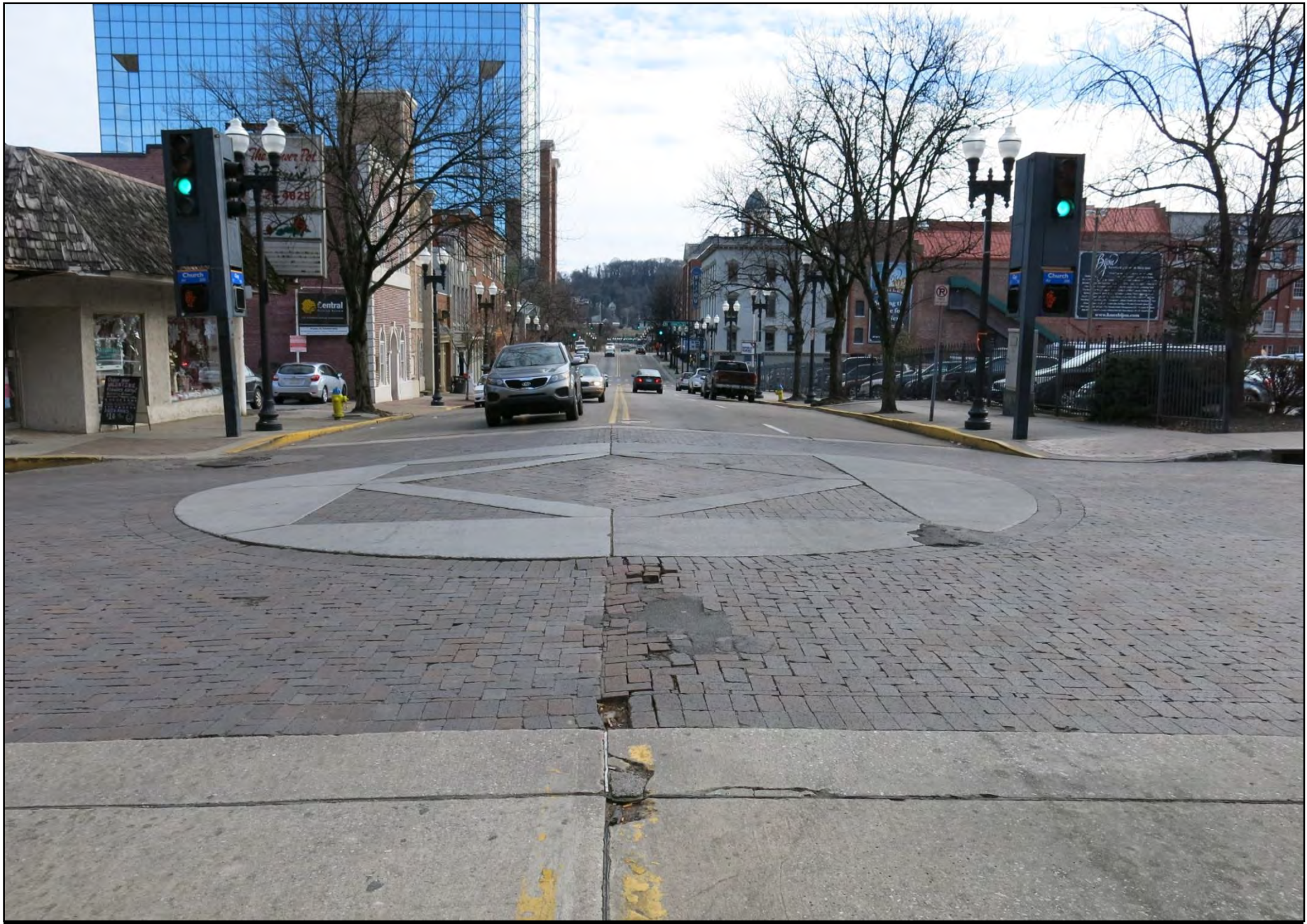
EXISTING CONDITIONS – GAY @ CHURCH
