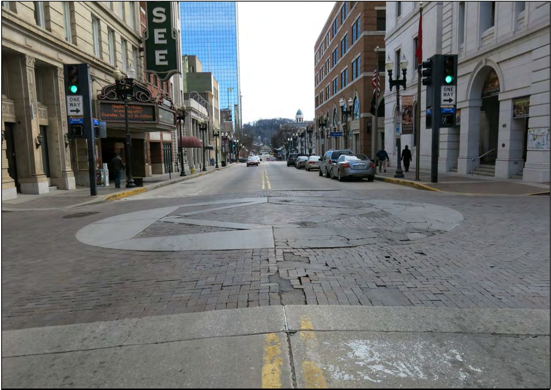
EXISTING CONDITIONS – GAY @ CLINCH
