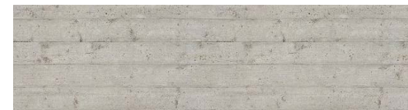
BOARD FORM CONCRETE
