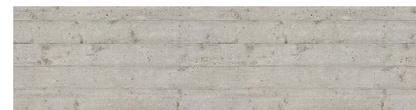
BOARD FORM CONCRETE
