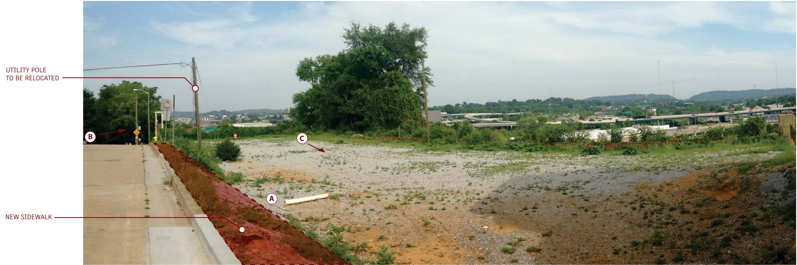
VIEW FROM SOUTHEAST CORNER
