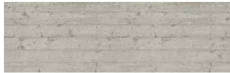
BOARD FORM CONCRETE
