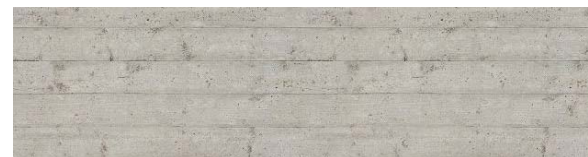
BOARD FORM CONCRETE
