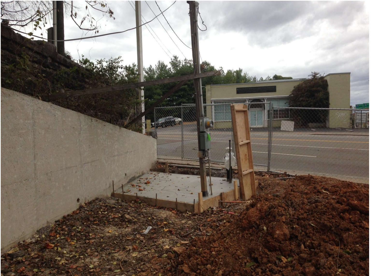
Concrete pad for chiller, adjacent to the Broadway sidewalk.
