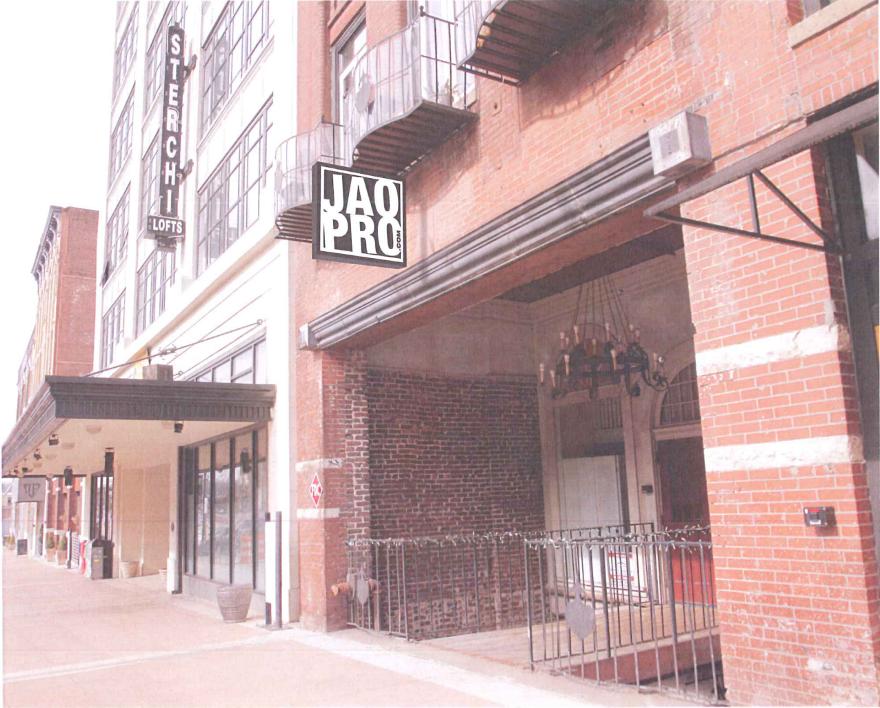
120 South Gay Street Exterior
