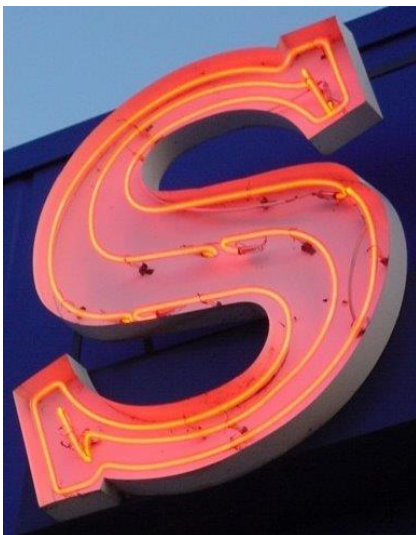
Typical open faced, metal, pan channel letter with red neon, for Sign 'A' and Sign 'B'
