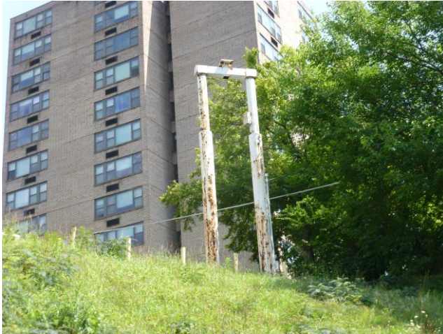
Existing pole location at top of hill above
