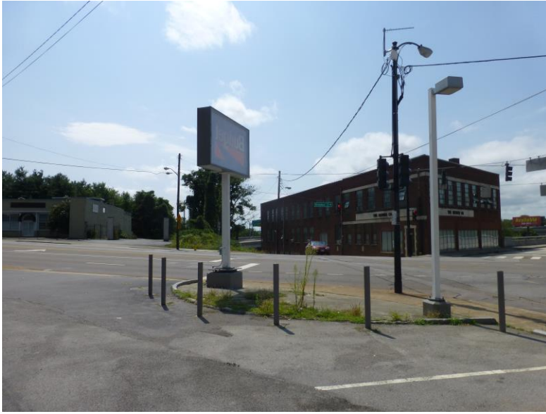
Existing pole sign location at intersection
