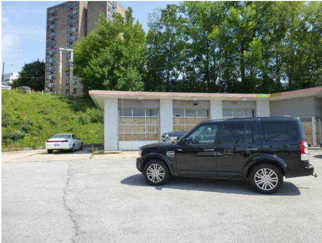
Existing location on top of garage bays
