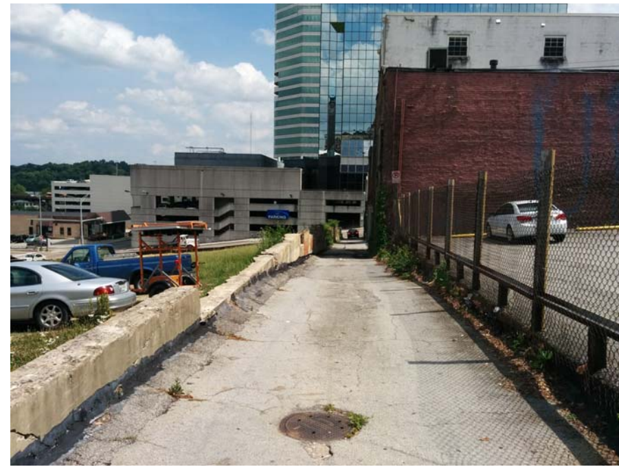
View looking down existing alley
