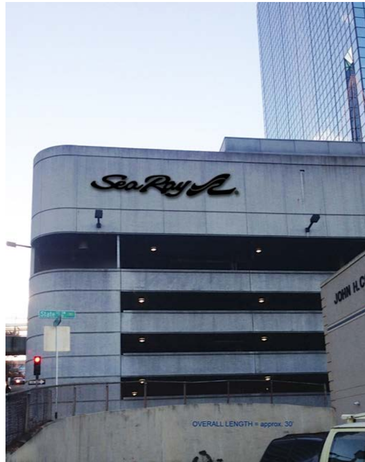
1 st Tennessee Parking Garage State Street
