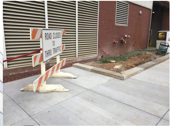
1 The landscaping beds/walls were cut back to accommodate the new rounded stairs.
