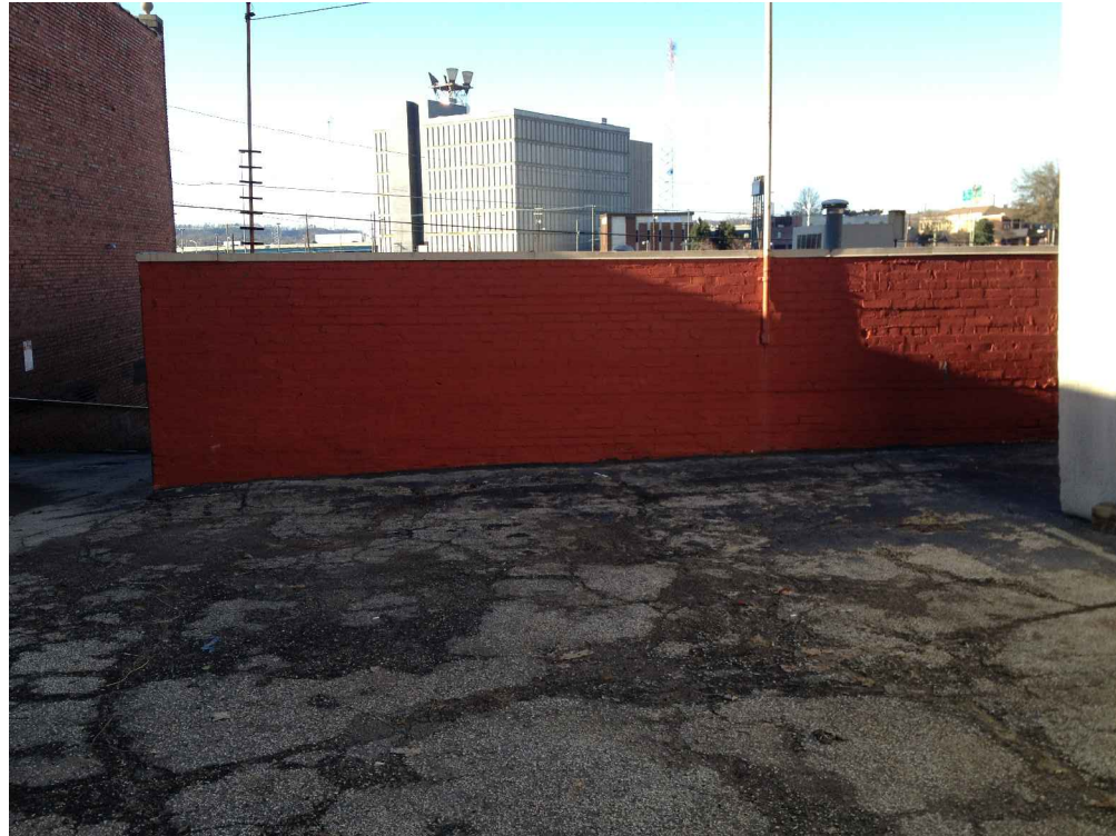
VIEW @ REAR OF EXISTING BUILDING
