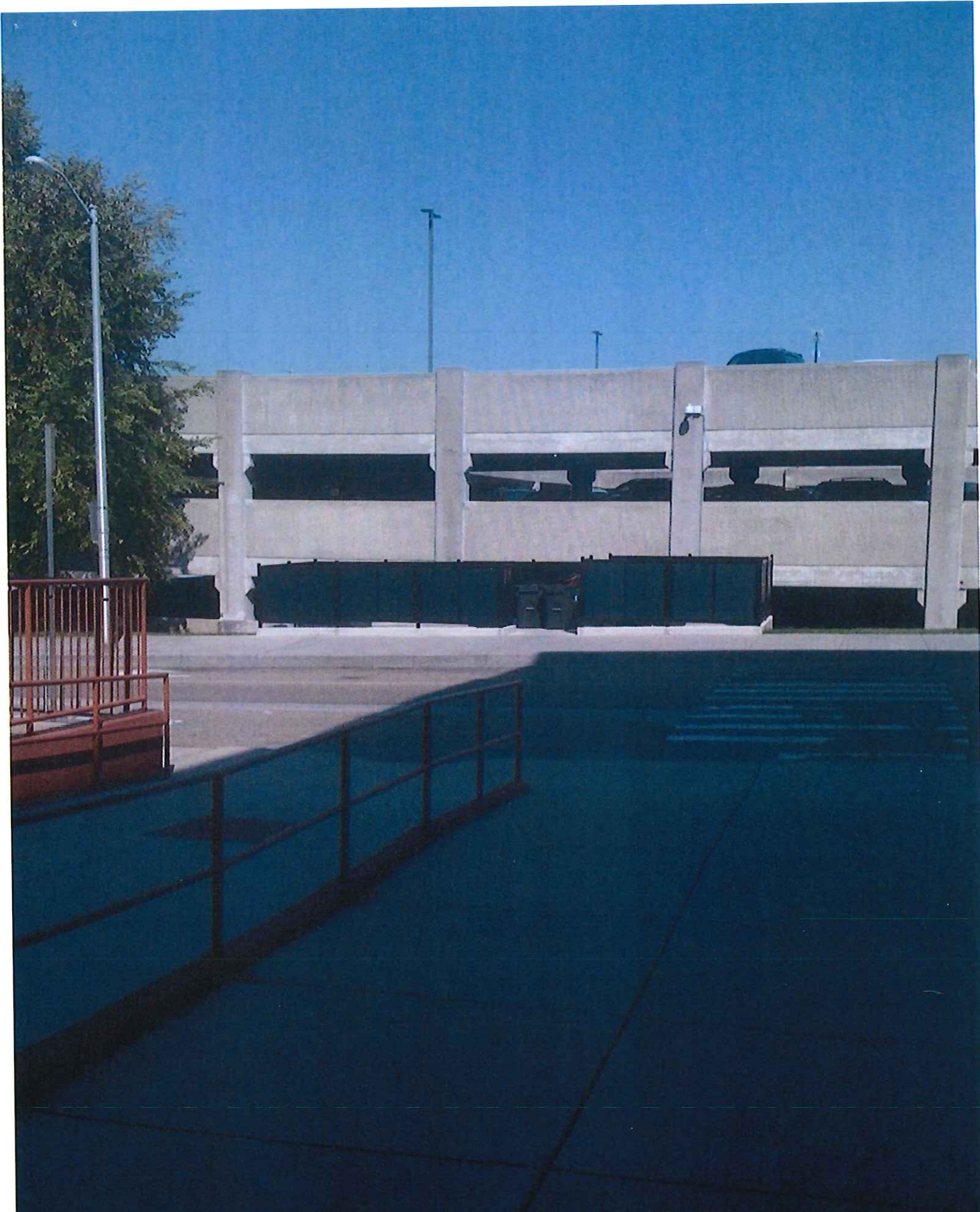
State Street Garage
