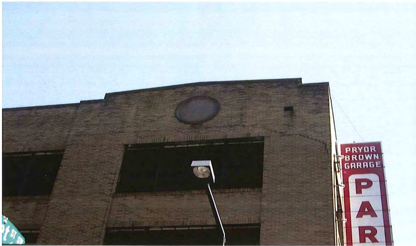
PRYOR BROWN PARKING GARAGE – EXTERIOR
