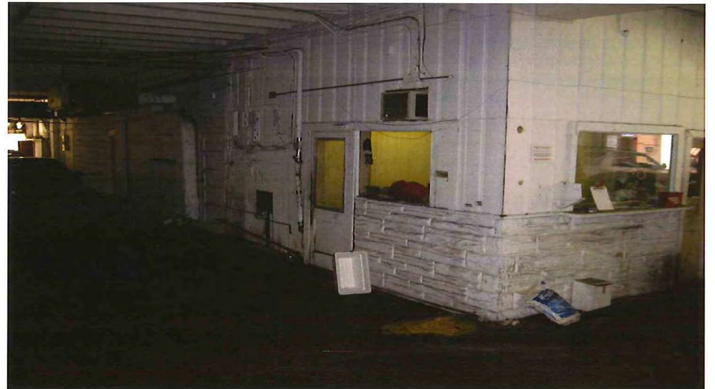
PRYOR BROWN PARKING GARAGE – MAN LIFT AND TENANT SPACES
