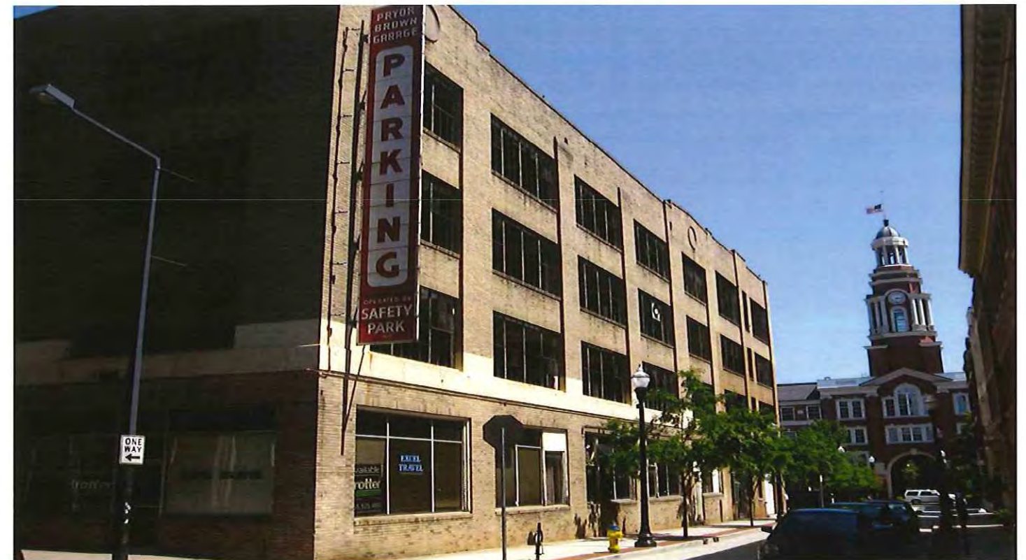
PRYOR BROWN PARKING GARAGE – EXTERIOR
