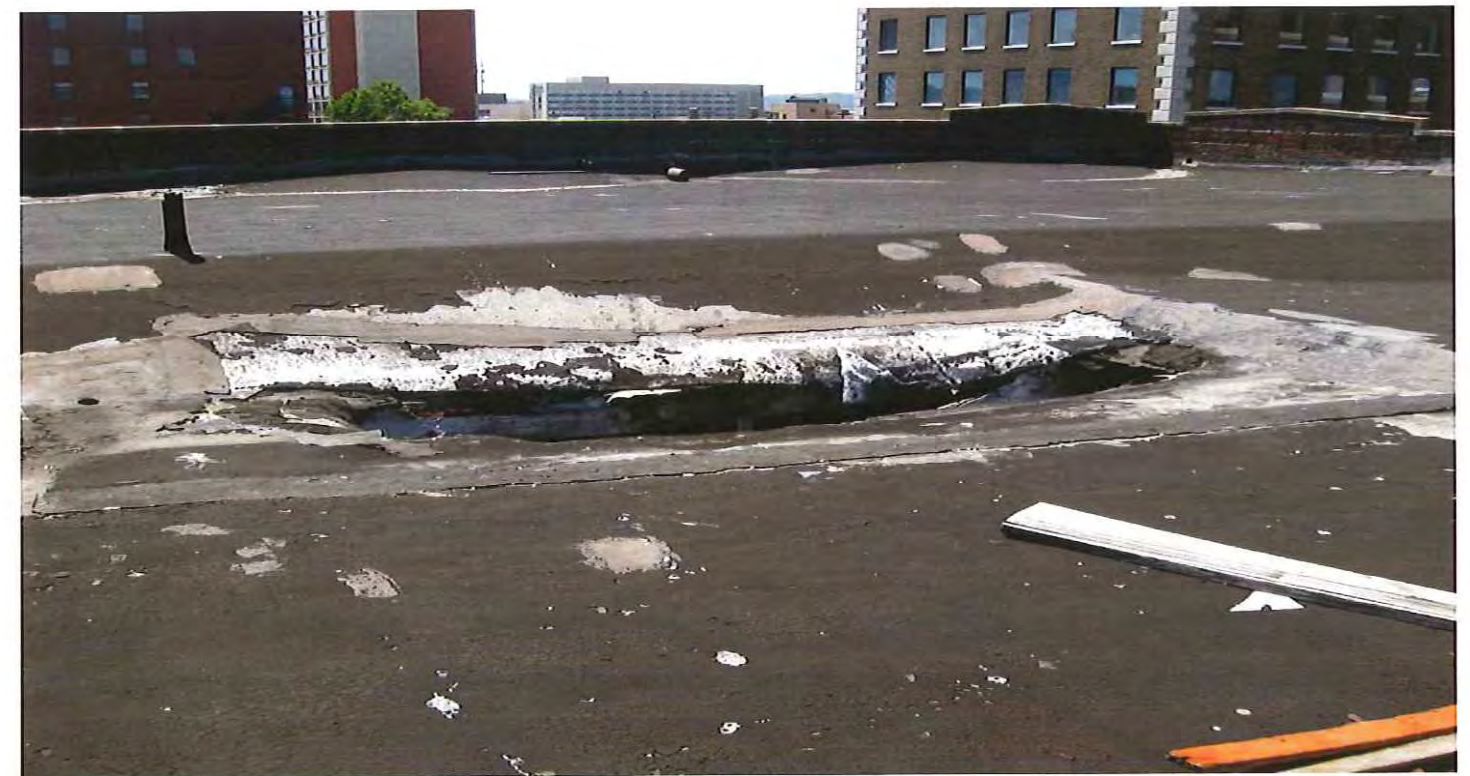
PRYOR BROWN PARKING GARAGE - ROOF
