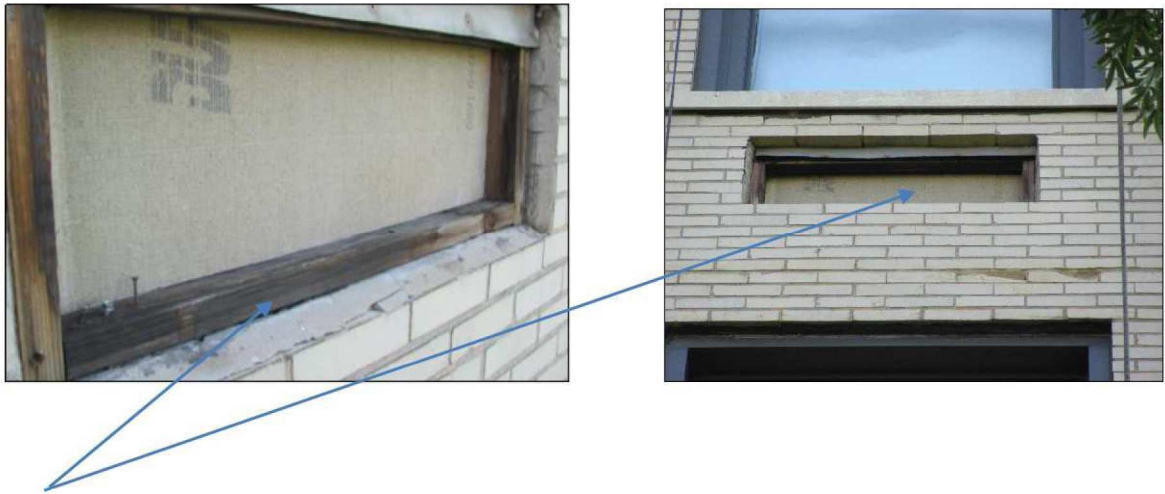
HVAC VENT OPENINGS TO BE BRICKED UP
