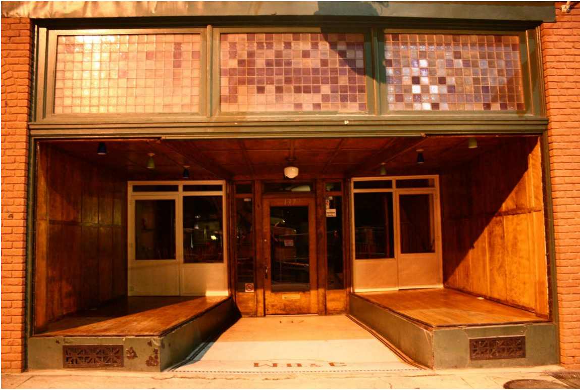
STOREFRONT AFTER DAMAGE
