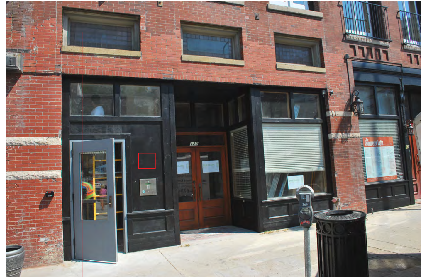
122 SOUTH GAY STREET FACADE
