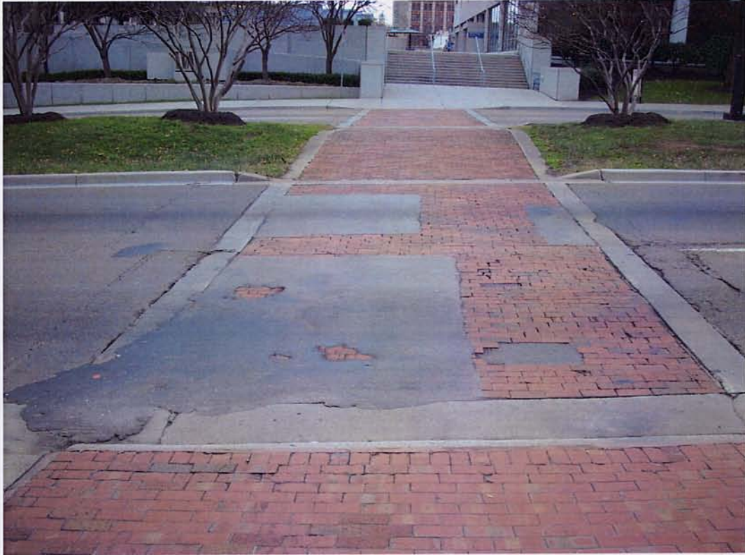
Existing Crosswalk at Summit Hill
