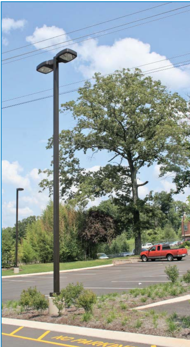
An example of cut-off fixtures on light poles that meet the requirements of the Design Guidelines
